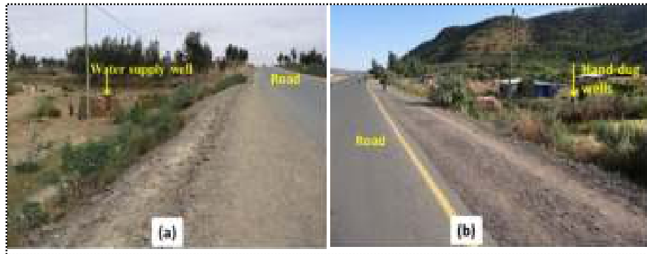
Plate 10. Upgrading of the road has resulted in an increase in groundwater availability due to recharge along roads in northern Ethiopia: (a) well at downstream of road, and (b) well at upstream of the road.
