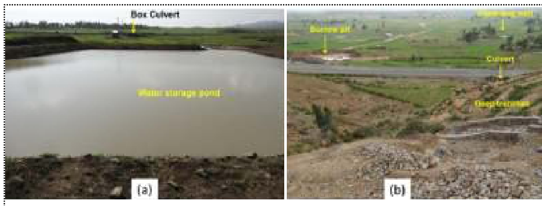
Plate 1. Use of ponds to harvest water from roads in northern Ethiopia: (a) excavated ponds, and (b) borrow pit converted into water storage in Tigray, Ethiopia.
