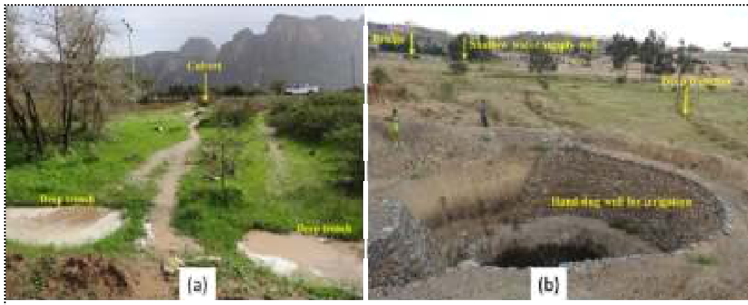
Plate 2. Water from roads (culverts, bridges) is channeled into series of deep trenches for enhancing soil moisture, reducing flooding and recharging groundwater in Ethiopia: (a) water from a culvert channeled into a deep trench, and (b) water from a bridge is channeled into series of deep trenches for enhancing shallow groundwater (for water supply and irrigation use).
