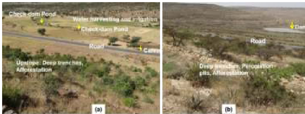
Plate 12. Example of a landscape continuum based land-water and infrastructure developments in Tigray, Ethiopia: (a) water from roads harvesting in check-dam ponds groundwater recharge and irrigation, (b) dam is saved from siltation due to land management at upslope and downslope of the road.
