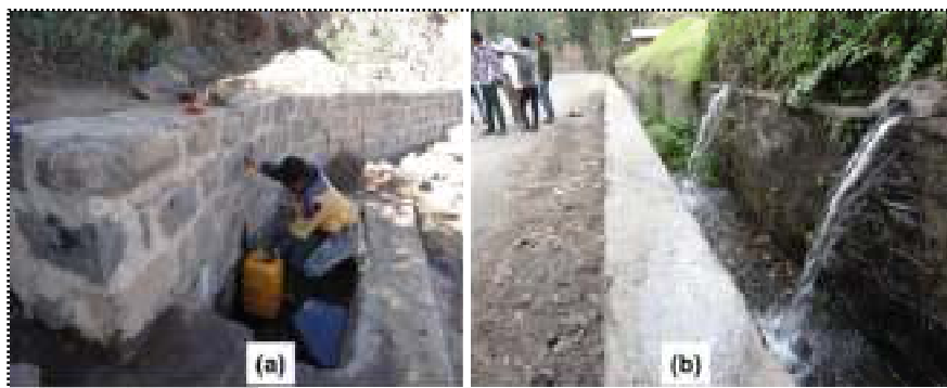
Plate 11. Spring developed from a road cut in northern Ethiopia: (a) for rural water supply, and (b) for small-scale irrigation purpose.
