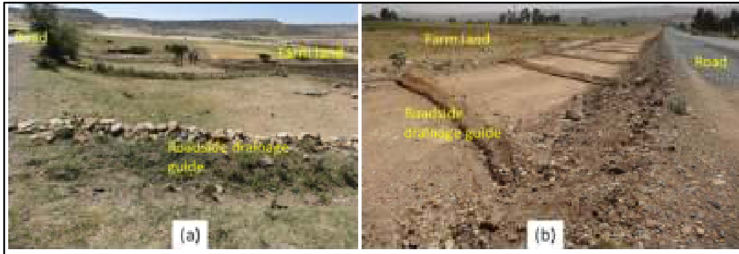
Plate 6. Road side runoff guided into farm lands as part of moisture conservation in northern Ethiopia: (a) runoff guide with stone bunds, and (b) runoff guide with earth bunds.
