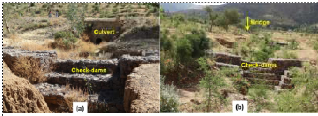
Plate 4. Use of gabion check-dams to manage water from roads in northern Ethiopia: (a) channeling water from a pipe culvert into a gabion check-dam, and (b) channeling water from a bridge into series of gabion check-dams for groundwater recharge.
