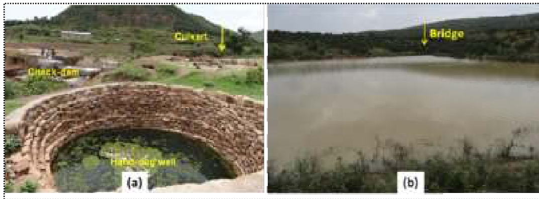
Plate 5. Water from road catchments is channeled into water storage structures for surface water harvesting and groundwater recharge in northern Ethiopia: (a) water from a culvert is stored in a check-dam pond, and (b) small dam is used to store water from a bridge.
