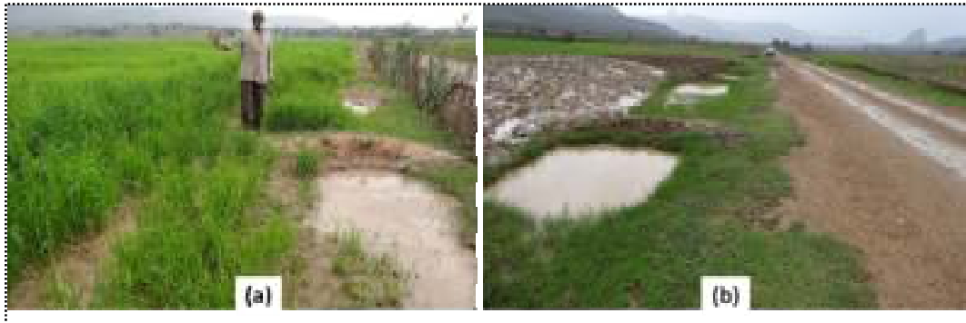
Plate 3. Use of roadside pits to enhance soil moisture and groundwater recharge in northern Ethiopia: (a) middle period of crop growth, and (b) early period crop growth.
