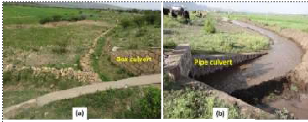
Plate 8. Roads used as dam embankments to store water and sediment in northern Ethiopia: (a) pond used to store sediment (used for sand mining) and water storage (for multiple use including groundwater recharge, surface water storage, etc), and (b) pond used to store water for small-scale irrigation and groundwater recharge.
